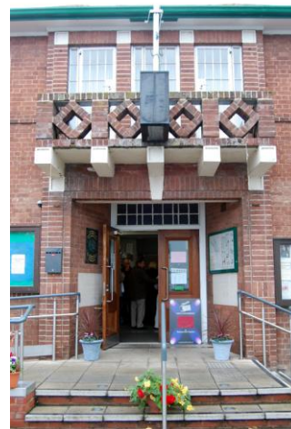
Topsham's Matthews Hall
