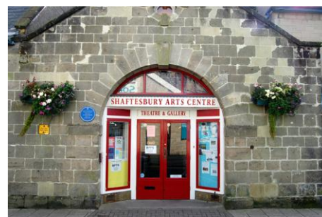
The 'new' Shaftesbury Arts Centre
